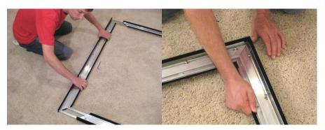
**Check Alignment, then Tighten Screws.** Confirming with your fingers that the joints are aligned nicely, go ahead and tighten the remaining set screws.
